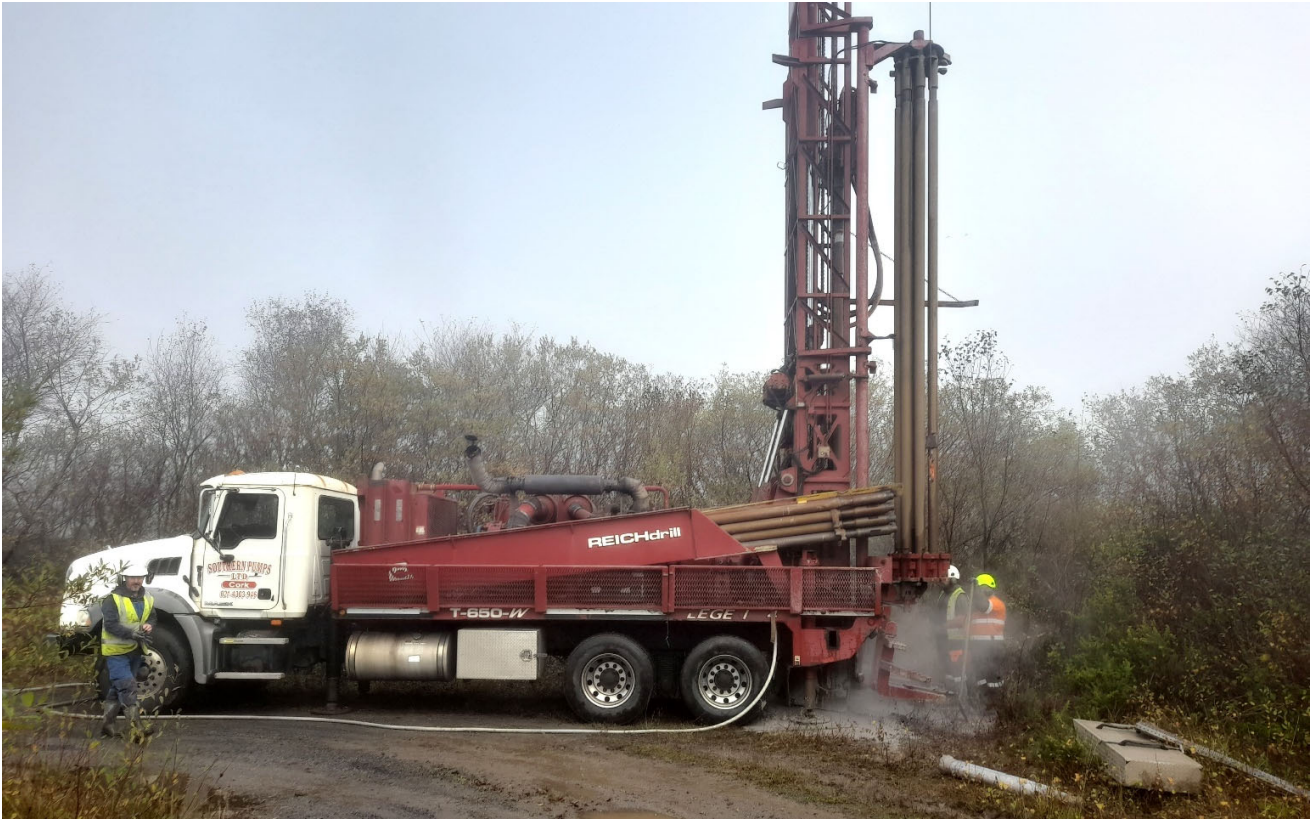
Photo 11: View of Southern Pumps drilling BH03 to the north of the Phase 2 expansion area.
