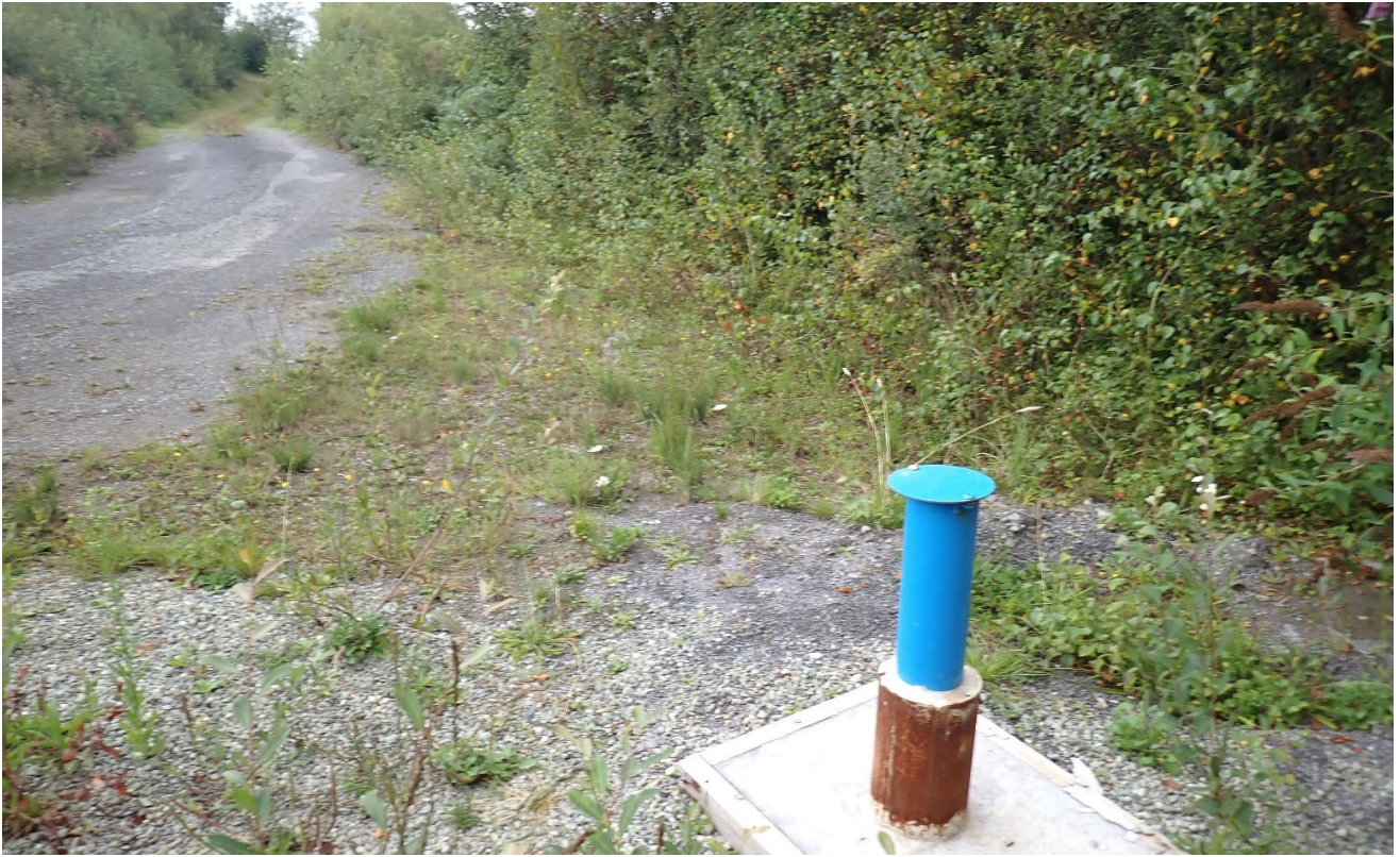
Photo 03: View West of the BH03 Headworks by the existing quarry track. (Tuesday 19 th Aug 2025).
