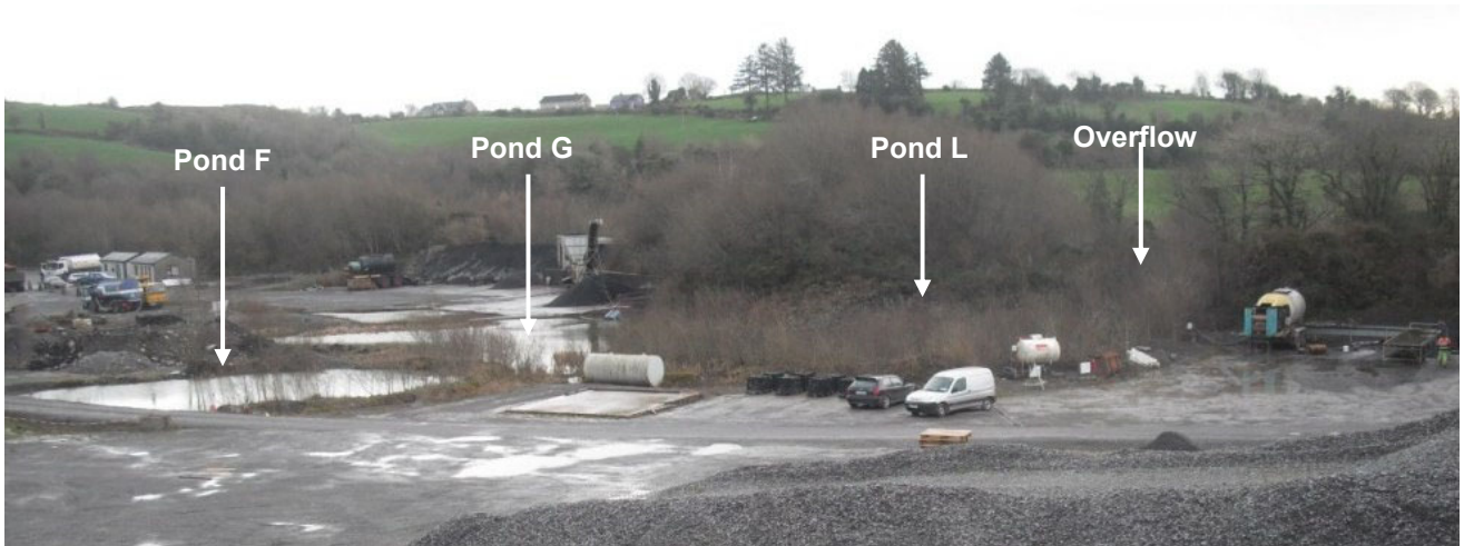
Photo 7.3.12: Old photo of view SE over lower part of Catchment Area A3 with Ponds F & G visible. Pond L is in overgrown area behind the white van and overflows south to the boundary stream.
