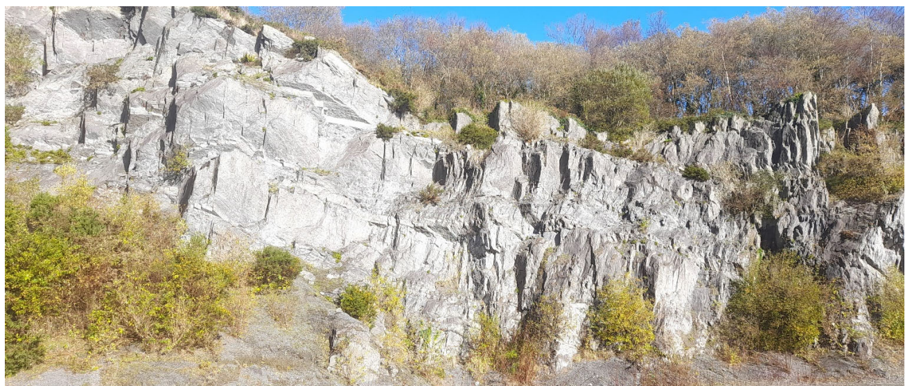
Photo 06: View north of second (northern) bench of old quarry which is part of Phase 1 Expansion area.
