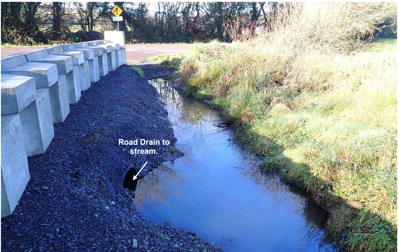
Photo 7.3.22: View of separate drainage ditch near the site access that takes road runoff and pipes it under the road to the local stream. This drain is not connected to the quarry area.
