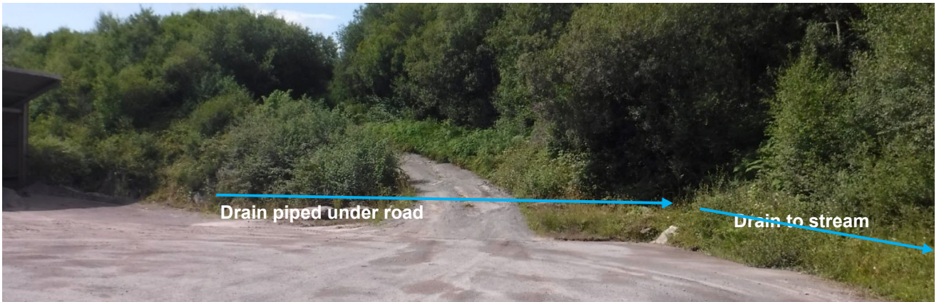
Photo 7.3.05: View NW of track going to the upper north side of site. Catchment Area A2. Yard & road drainage goes to the stream here, at a point just above the sites discharge Location 02.
