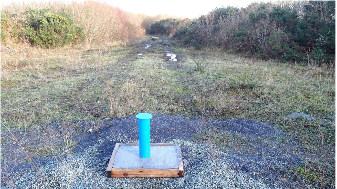
Photo 16: View East of BH05 headworks, in the NW corner of the site, at the end of the internal track. (This BH was not sampled as part of the initial GW sampling works as the track was too wet to drive on.)
