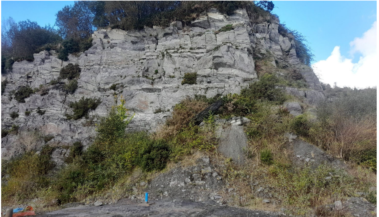
Photo 07: View north across west side of the tarmac site with old quarry face in background.
