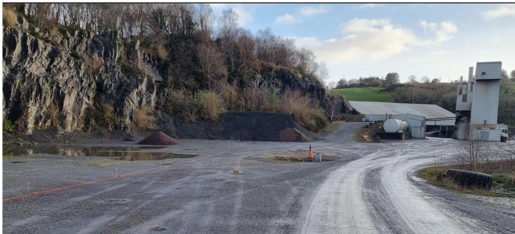
Figure 2.1C. Plant area and previously worked face looking east
