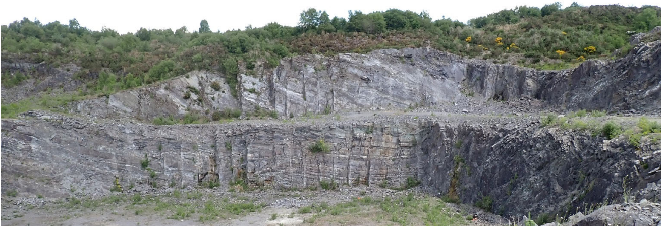
Photo 02: View north of existing double benched quarry high wall of 2014 quarry face. Proposed Phase 3.
